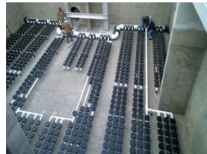
New Fine Bubble Diffusers
