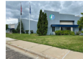
Cedar Avenue truck station Photo from Mark Moenlenbrock, MnDOT
