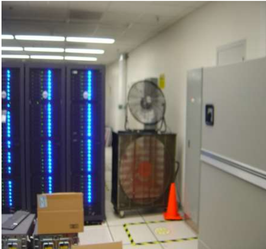
Fans were used to redirect air
