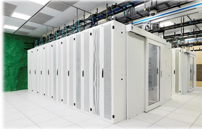
Cold aisle containment at WPA-1
