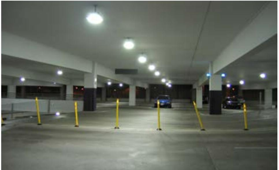
High-efficiency lighting from fluorescent, induction, and LED sources could offer immediate returns without requiring major changes to parking structures, such as the one pictured above. A BBA project team studied the lighting technology to create a performance specification.
