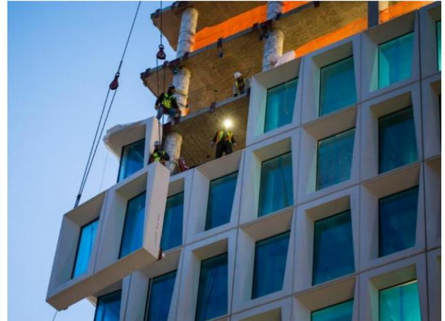
Construction workers installing an energy efficient prefabricated building envelope. Source: U.S. Department of Energy.
