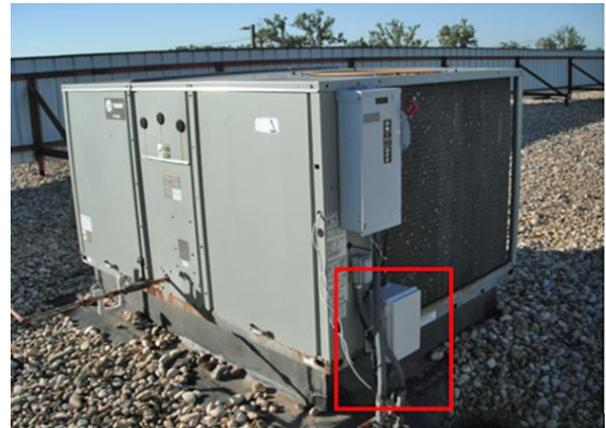
12.5-ton, two-stage RTU at an office building in Beltsville, MD, after installing the Hardware SMDS (outlined in red)
