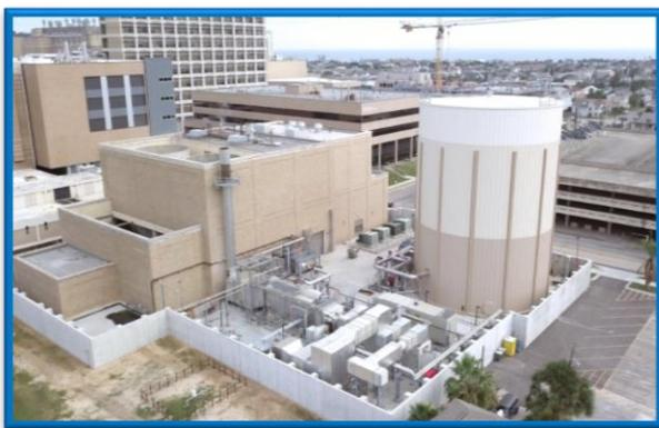
*University of Texas Medical Branch CHP System with installed floodwalls. Photo courtesy of UTMB Health*
