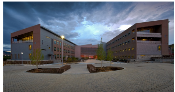
Figure 1. NREL's Research Support Facility. Image courtesy of Dennis Schroeder.
