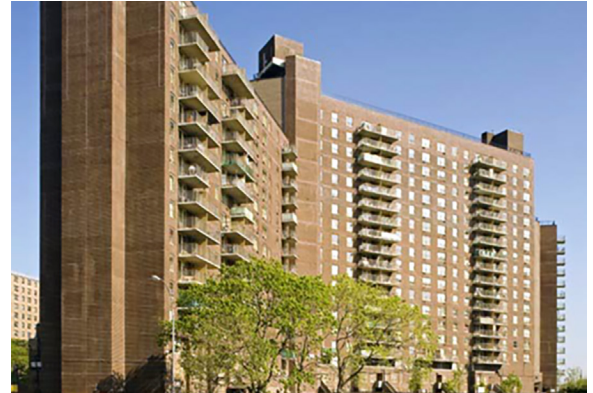
The Sea Park apartment complex in Brooklyn, New York, installed 300 kW of CHP to reduce costs through energy efficiency improvements. CHP provides approximately 1/4 of the buildings' electricity needs. Photo courtesy of U.S. Department of Energy (DOE) New York-New Jersey CHP Technical Assistance Partnership (CHP TAP).
