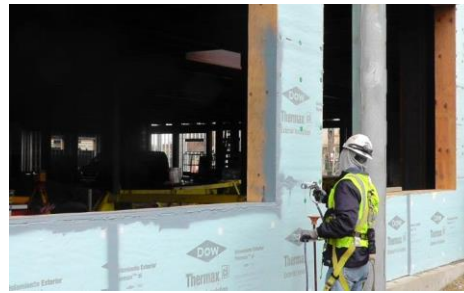
Figure 4. LIQUIDARMOR™ CM sprayed over board joints and a window rough opening.
