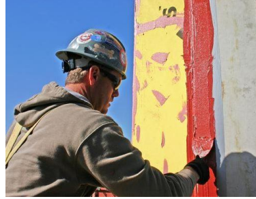
Figure 3. Liquid flashing applied with a caulk gun and trowel.
