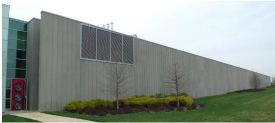
Figure 6. Back of the Homeland Security Training Center. Exterior walls are made of insulated precast concrete panels.
