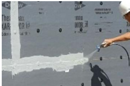
Figure 4. LIQUIDARMOR™ CM sprayed over board joints and a window rough opening.
