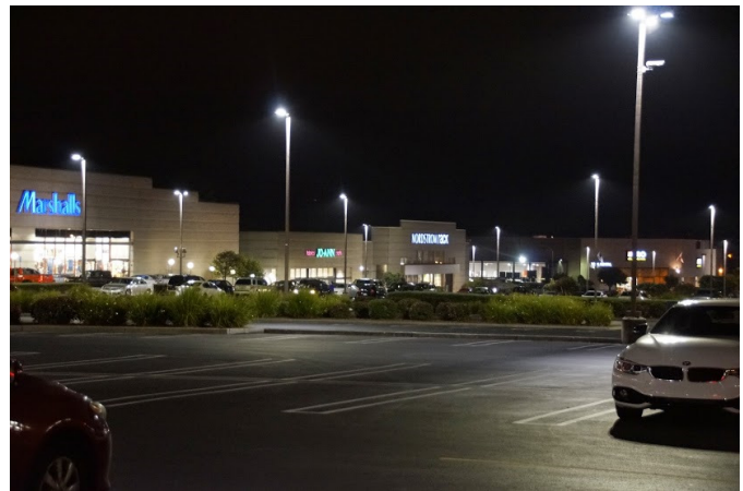
280 Metro Center in Colma, CA. Image courtesy of Kimco.
