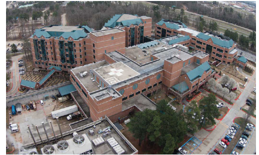
St. Michael Hospital in Texarkana, Texas, was included in a larger lighting retrofit where 16,400 troffers were retrofitted with LED lighting to achieve a 58% reduction in energy use. Photo courtesy of CHRISTUS Health.
