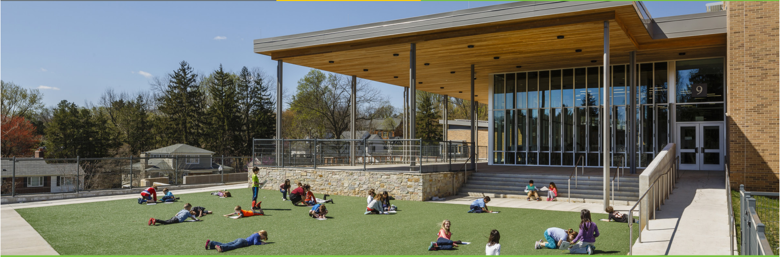
At Discovery Elementary, a zero energy school in Arlington, Virginia, the architect used building orientation and shading to maximize daylighting while minimizing heat gain. Photo from VMDO Architects/©Lincoln Barbour
