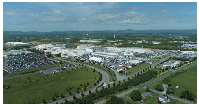
Volvo New River Valley facility. Photo credit: Volvo Group North America.
