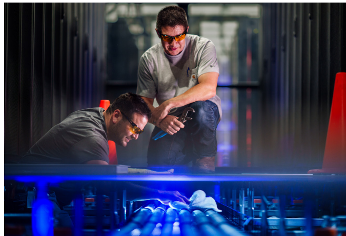
Manuel Torres, left, and Tony Tafoya check the liquid cooling system in Sandia's high-performance computing building. Photo by Craig Fritz/Sandia National Labs Courtesy of Craig Fritz, Sandia National Laboratories Corporate Journalist
