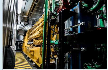
The Rimco Cat CG170-20 generator is providing 2 MW of power to the processing facility and warehouse.
