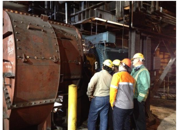
Participants at an In-Plant Training use a strobe tachometer to determine the rotational speed of a combustion air fan motor.
