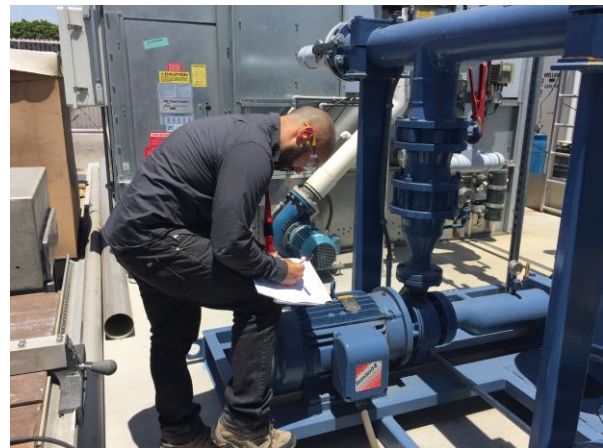
An Industrial Assessment Center (IAC) student examines pumps at an industrial facility. Photo courtesy of the San Francisco State University IAC.
