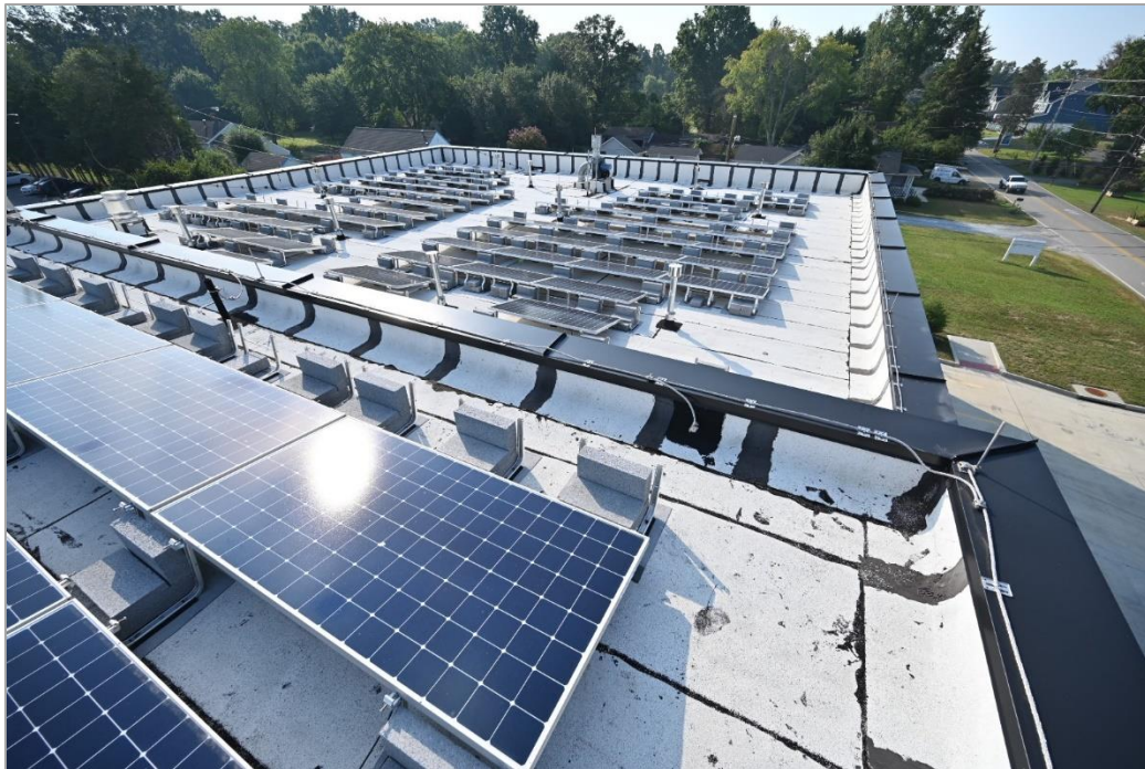
Woodlawn Fire Station
