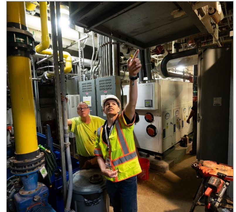
Reston Community Center Heating System Upgrade
