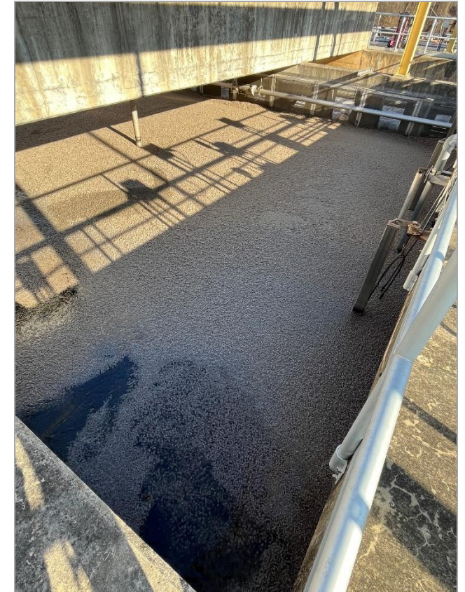
Moving Bed Biofilm Reactor at the Noman Cole Water Recycling Facility
