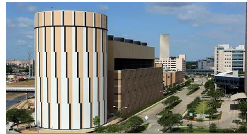
This 8.8-million-gallon chilled-water TES tank provides 75,000 ton-hours of cooling, integrated with 45 MW CHP at Texas Medical Center in Houston. 2 Photo courtesy of TECO
