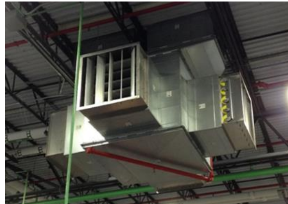
Discharge Head with Minimal Ductwork
