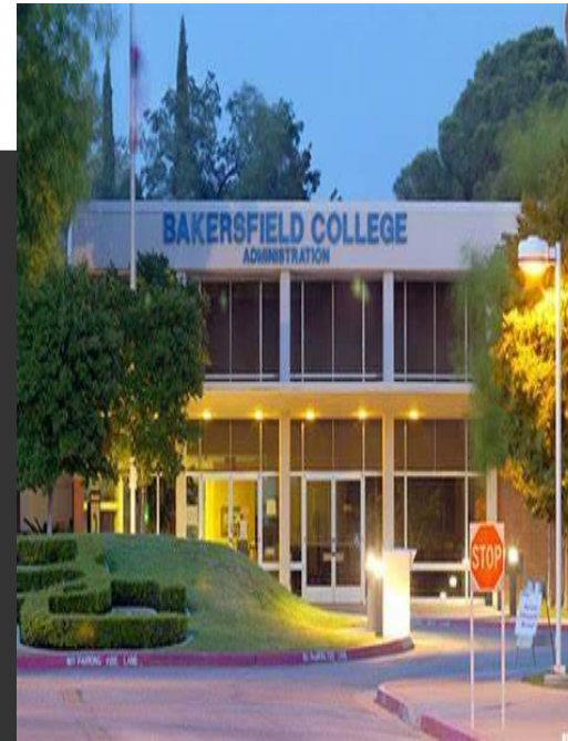
Complete Modernization Renovation
