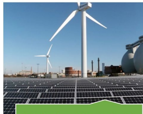
MWRA Deer Island solar PV and wind turbines
