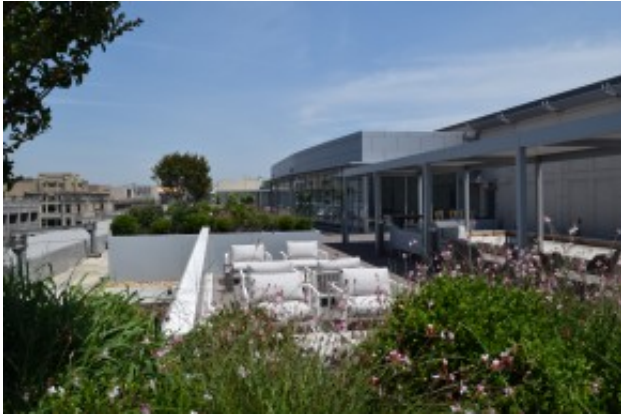
Rooftop of the District Center
