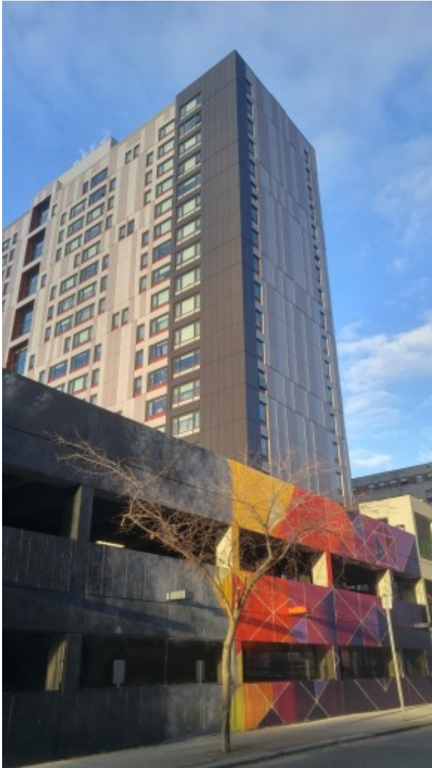
Exterior view of Manning Apartments post construction
