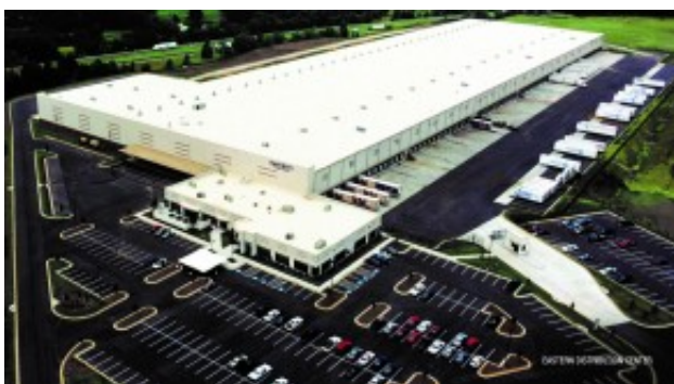
Havertys Eastern Distribution Center in Braselton, GA (overhead)
