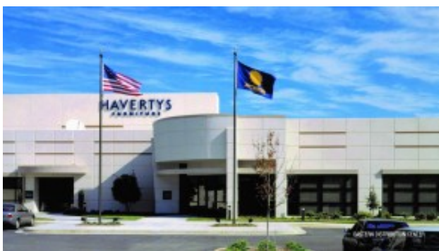
Havertys Eastern Distribution Center in Braselton, GA (front)
