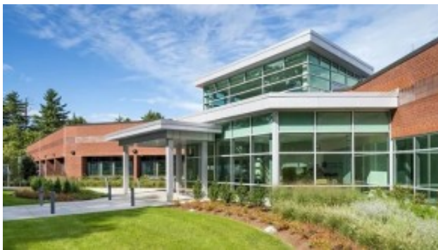
Outside view of Digital Realty's Bedford data center
