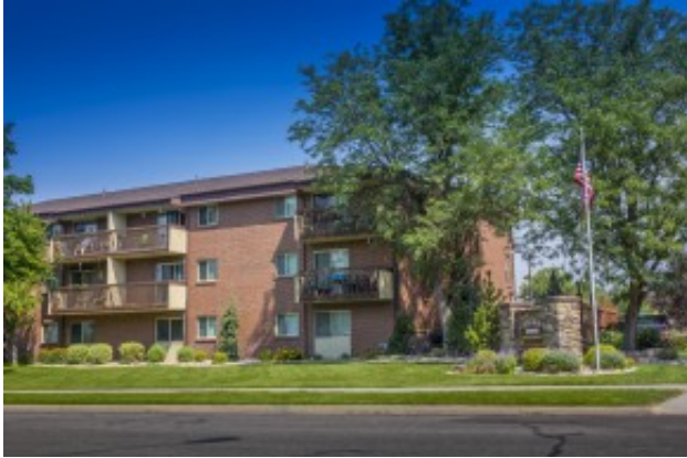
Rear view of units at Union Gardens
