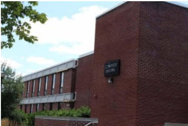
Computer Building Facade
