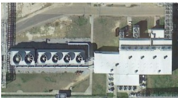
Canton, MS Utilities Plant (CUP)
