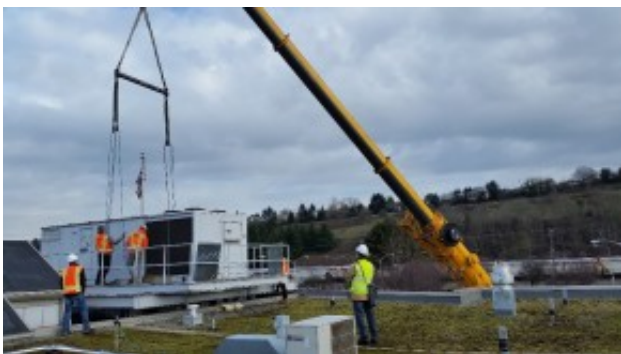
Removal of inefficient RTU
