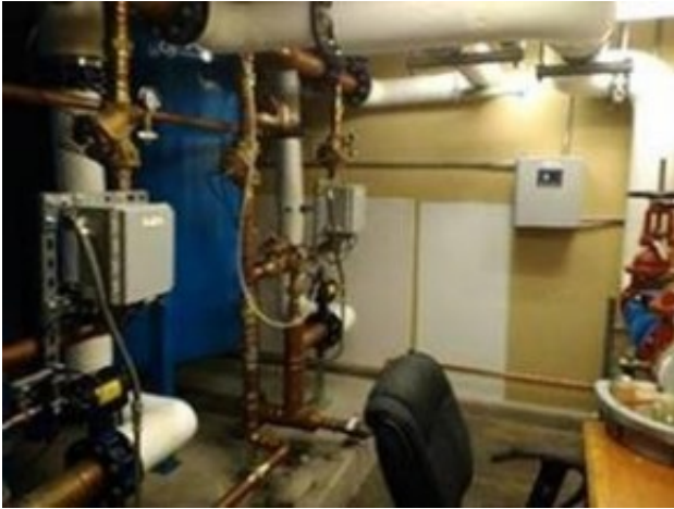
Water Softener Addition
