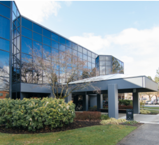
Main entrance, Nike Miler building
