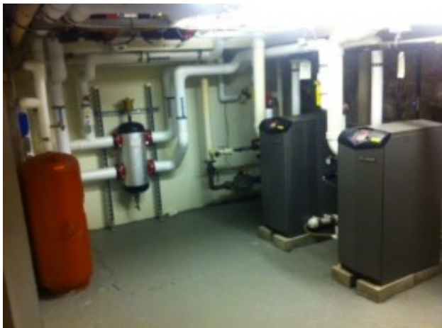
Cascap installed both energy and water efficient upgrades
