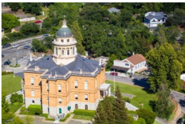
Auburn Courthouse aerial
