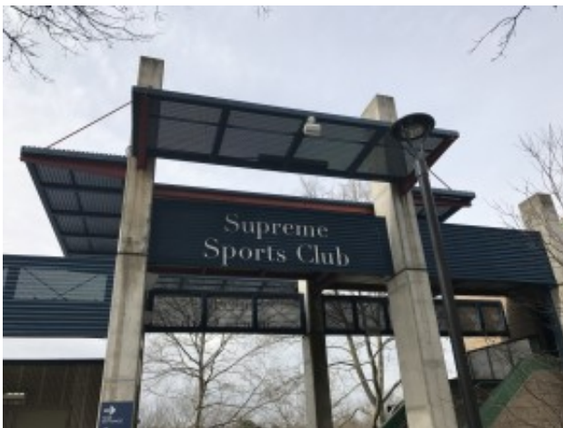
Main entrance with LED lighting.
