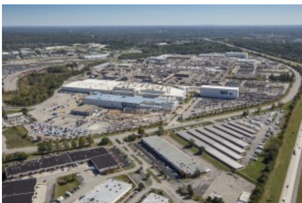
New Paint Shop Concept Under Construction
