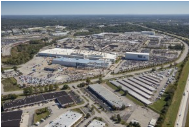
New Paint Shop Concept Under Construction
