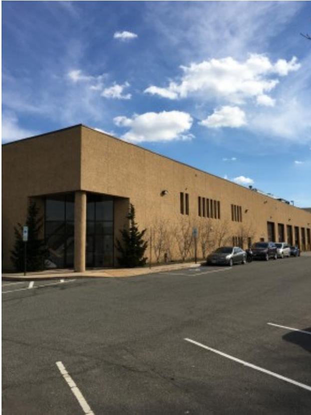
Equipment Bureau, Entrance
