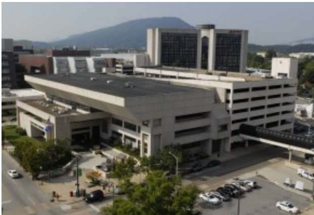
Exterior view, Chattanooga Public Library; iconic Lookout Mountain in background
