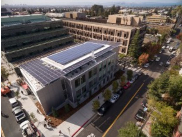
Rooftop Solar Array
