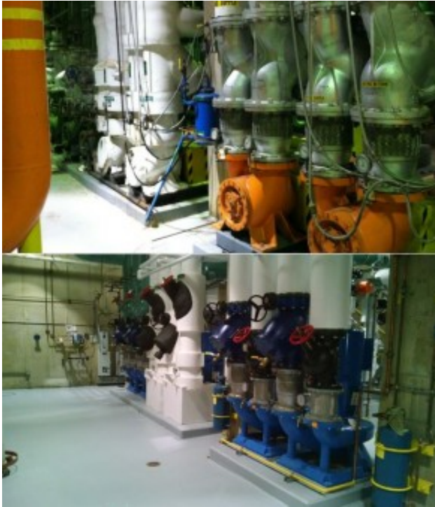
Before and After Pump Replacement
