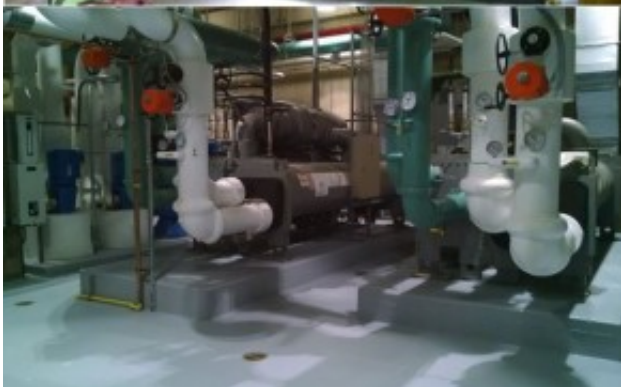
Before and After Chiller Replacement
