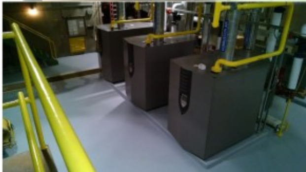
Before and After Boiler Replacement
