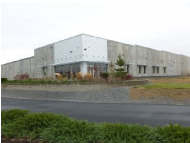
Intuit's Quincy, Washington Data Center
