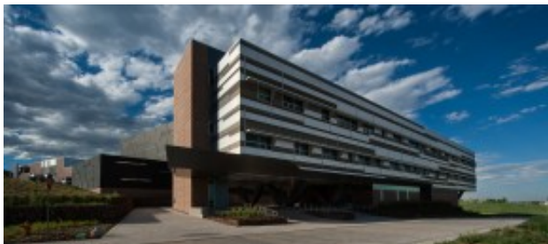
Energy Systems Integration Facility
