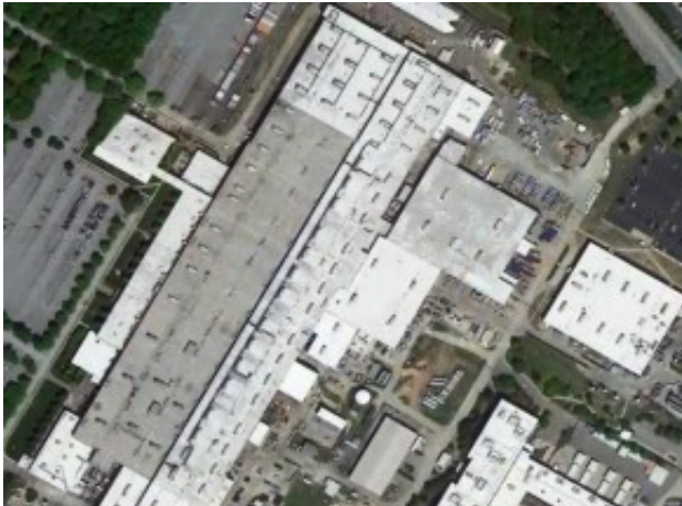
100 roof-mounted HVAC units, each the size of a small RV
