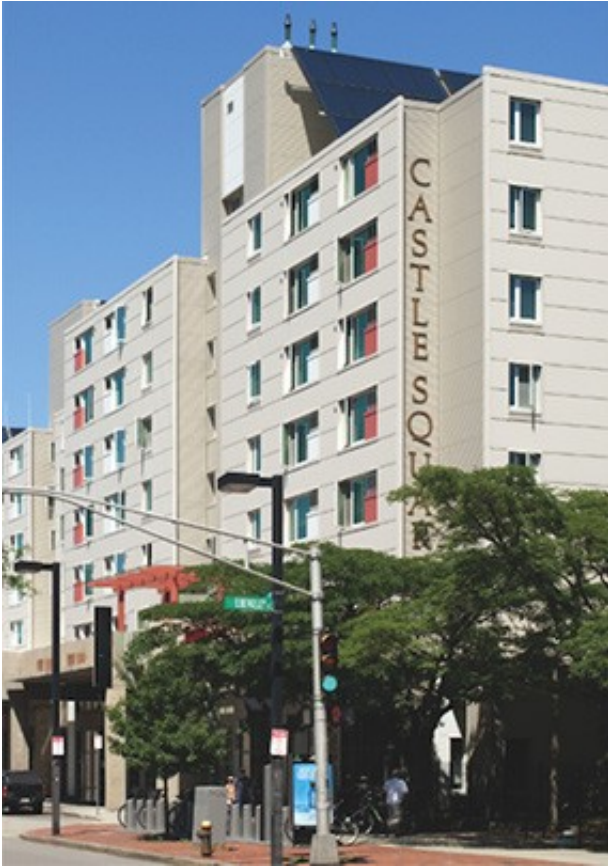
Post renovation with new facade
