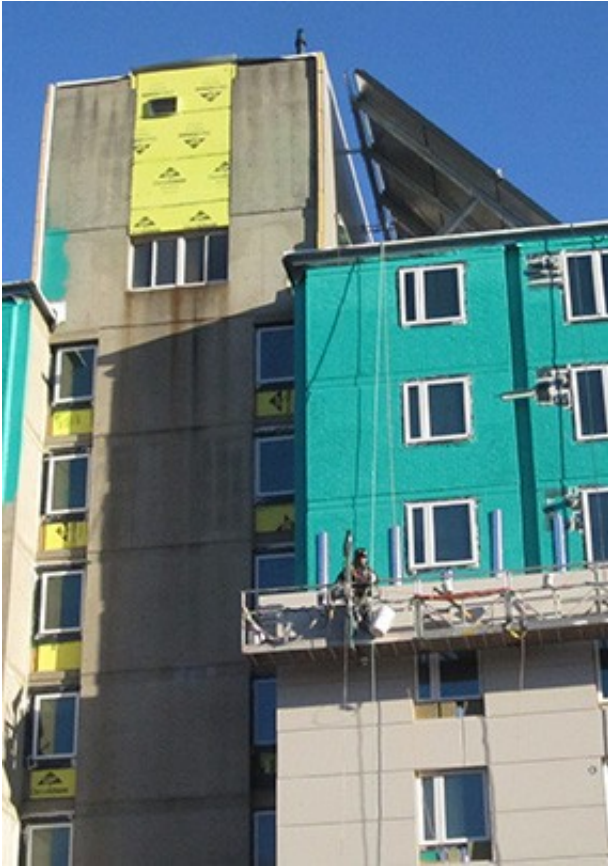
Applying exterior insulation and cladding
