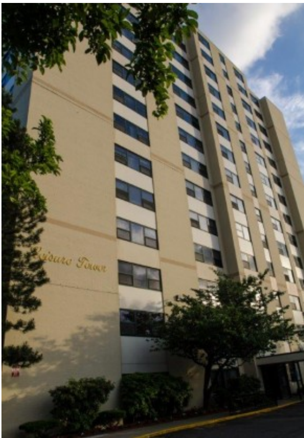
Exterior view of the Leisure Tower
