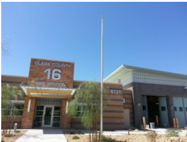
Street View of New Clark County Fire Station 16
