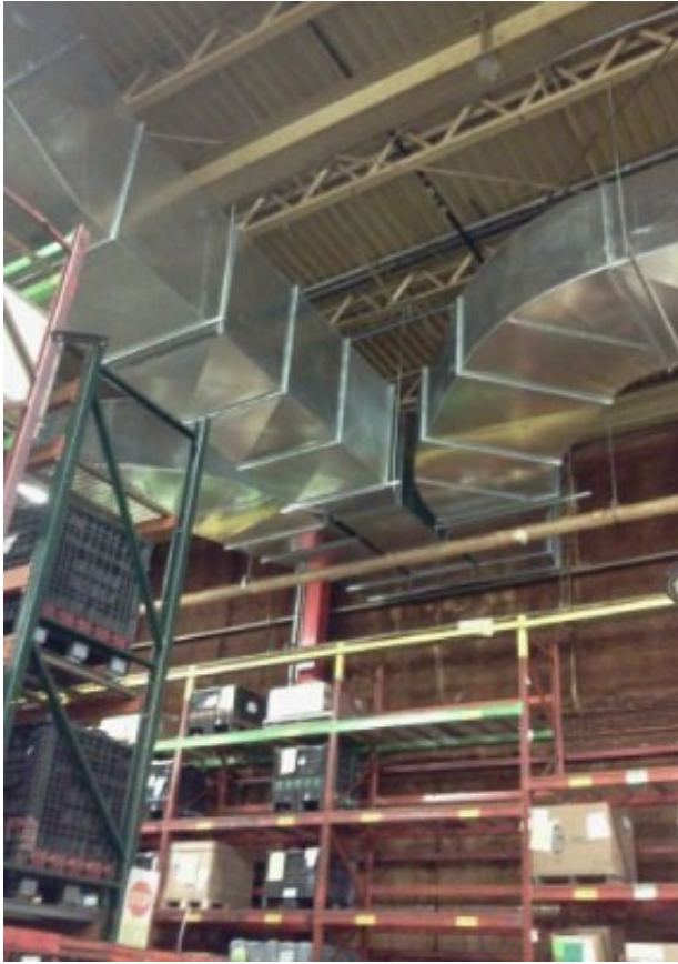
New duct work installed at the engine plant
