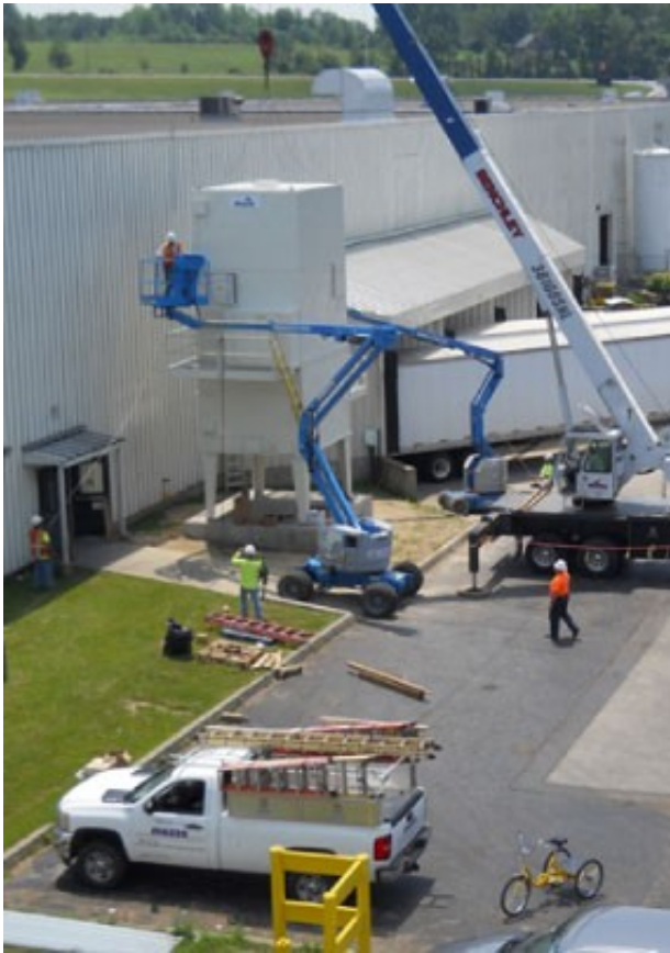
Workers installing air handlers outside plant
