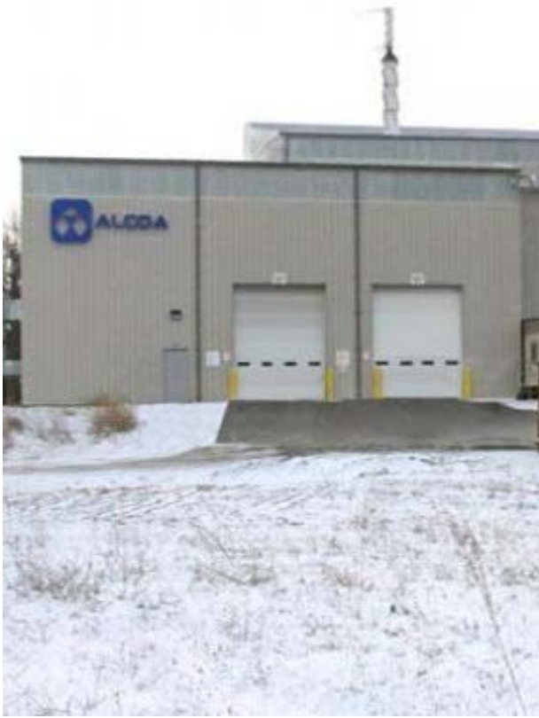
Exterior view of the casthouse
